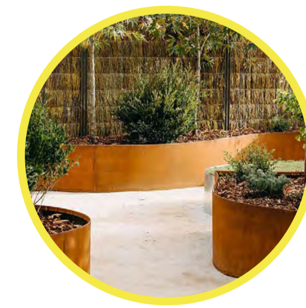
CORETEN WALL FOR INFORMAL RAISED GARDEN BEDS WITH THE POTENTIAL FOR CUSTOM SEATING. MINOR IMPLEMENTATION FOR SELECT AREAS ONLY
