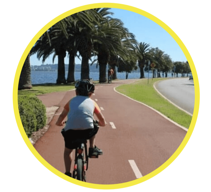
RED ASPHALT TRAFFICABLE DUAL USE PATH PRIMARYLY FOR PEDESTRIAN USE (ALLOWS FOR MAINTENANCE AC- CESS)
